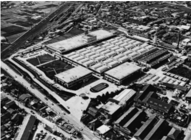
Aerial view of Takasaki Plant
