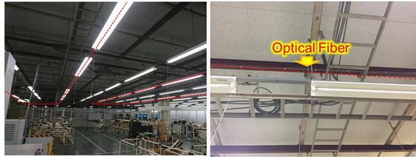
(a) Optical Fiber Lay Out in Factory Ceiling
