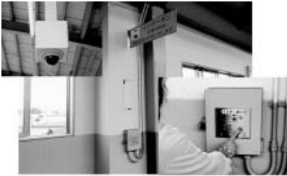
Photo 1 Scene depicting utilization on site: Camera and IP intercom inside the station.
