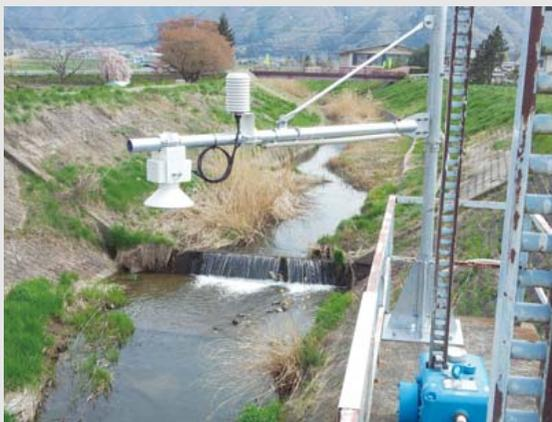
For one test bed site prepared by the National Institute of Information and Communication Technology (NICT), we developed and delivered a river monitoring system that enables remote monitoring of river water levels using a wireless 920 MHz band multi-hop network to collect data via sensors for tracking water levels and rainfall amounts.
