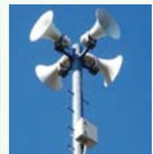
An all-weather 920MHz band wireless box installed on an existing outdoor loudspeaker system
