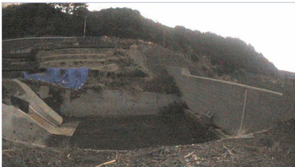
Photo 3. Landslide Barrier Monitoring (2:00am Image)
