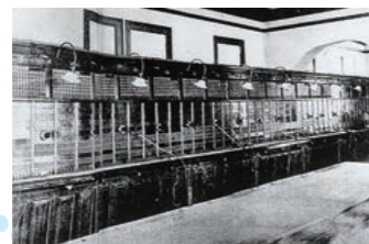
Magnetic parallel multiple telephone switchboard
