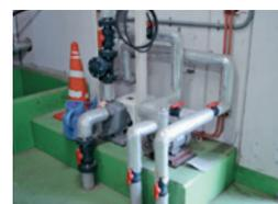
Pump to carry high-temperature drainage to snow shoveling pipes
