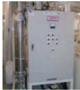
Cleansing treatment equipment for waste fluids of wafer cutting water
