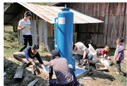
Installation of a drinking water filtration system
