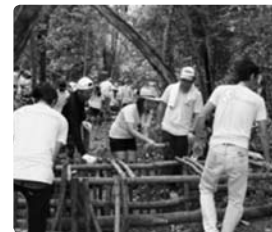
Employees installing water weir barrier
