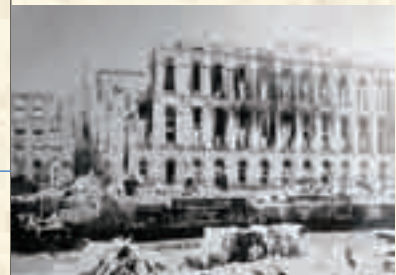
Kyobashi Telephone Office damaged by the Great Kanto Earthquake
