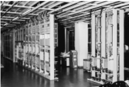
Model D10 electronic switching system (Yodobashi Telephone Office, Tokyo)
