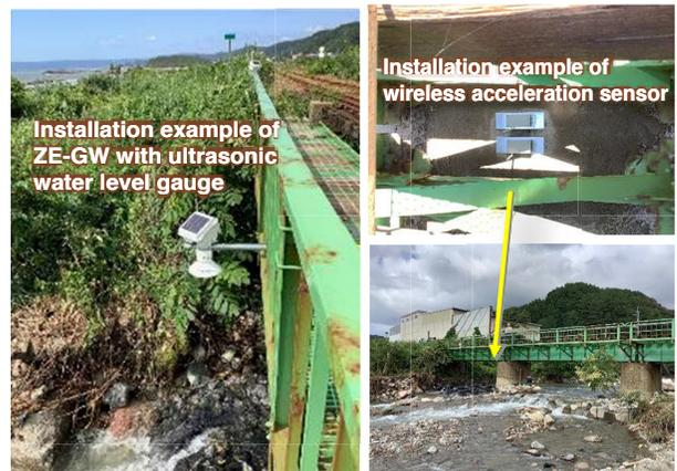
**Figure 3. Installation on Railway Bridge**
