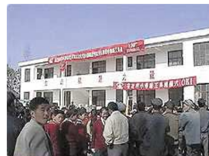
This new school house, in the PRC’s Shanxi province, was built with support from Oki.
