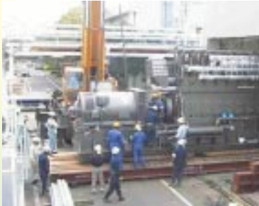
Construction of our semiconductor plant's cogeneration system was completed in fiscal 2001.
