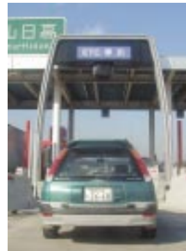
The ETC system is part of Oki's ITS service, enabling automatic toll transactions without the need to stop at the toll gate.
