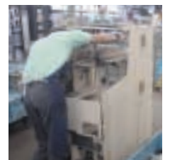
Dismantling work of ATM equipment
