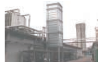
● A Chimney Refurbished for Noise Reduction (Example from Fiscal 2001)
