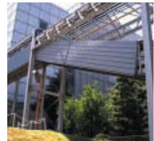
● Installation of Pipes above the Ground (Example from Fiscal 2001)
