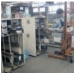
Disassembly of ATM into Large Parts
