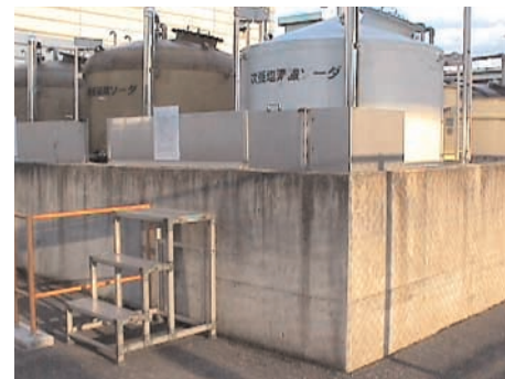
The concrete casing of a waste water processing tank
