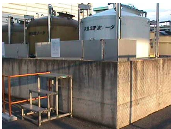
Concrete encasing the liquid waste processing tank (Tomioka area)
