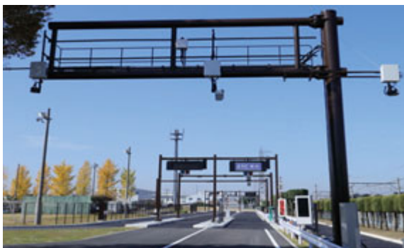
Photo 2. ITS Test Course
