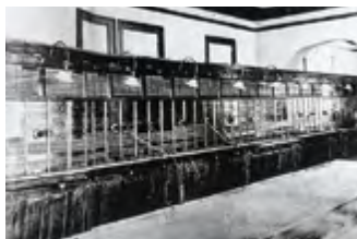
Magnetic parallel multiple telephone switchboard
