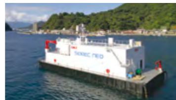
New "SEATEC NEO" Stationary Measurement Barge
